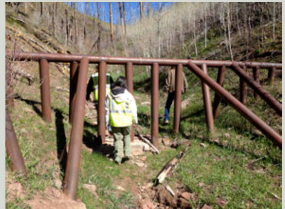
Debris rack at Lemon Dam
