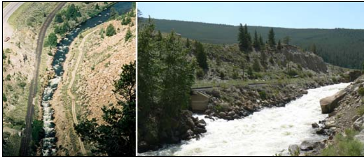
Figure 20—Granite Gorge Rapids at Pine Creek. Left: view upriver of start of rapids; Right: highwater 28 June 2008. Pine Creek flows from left through concrete railroad underpass.
