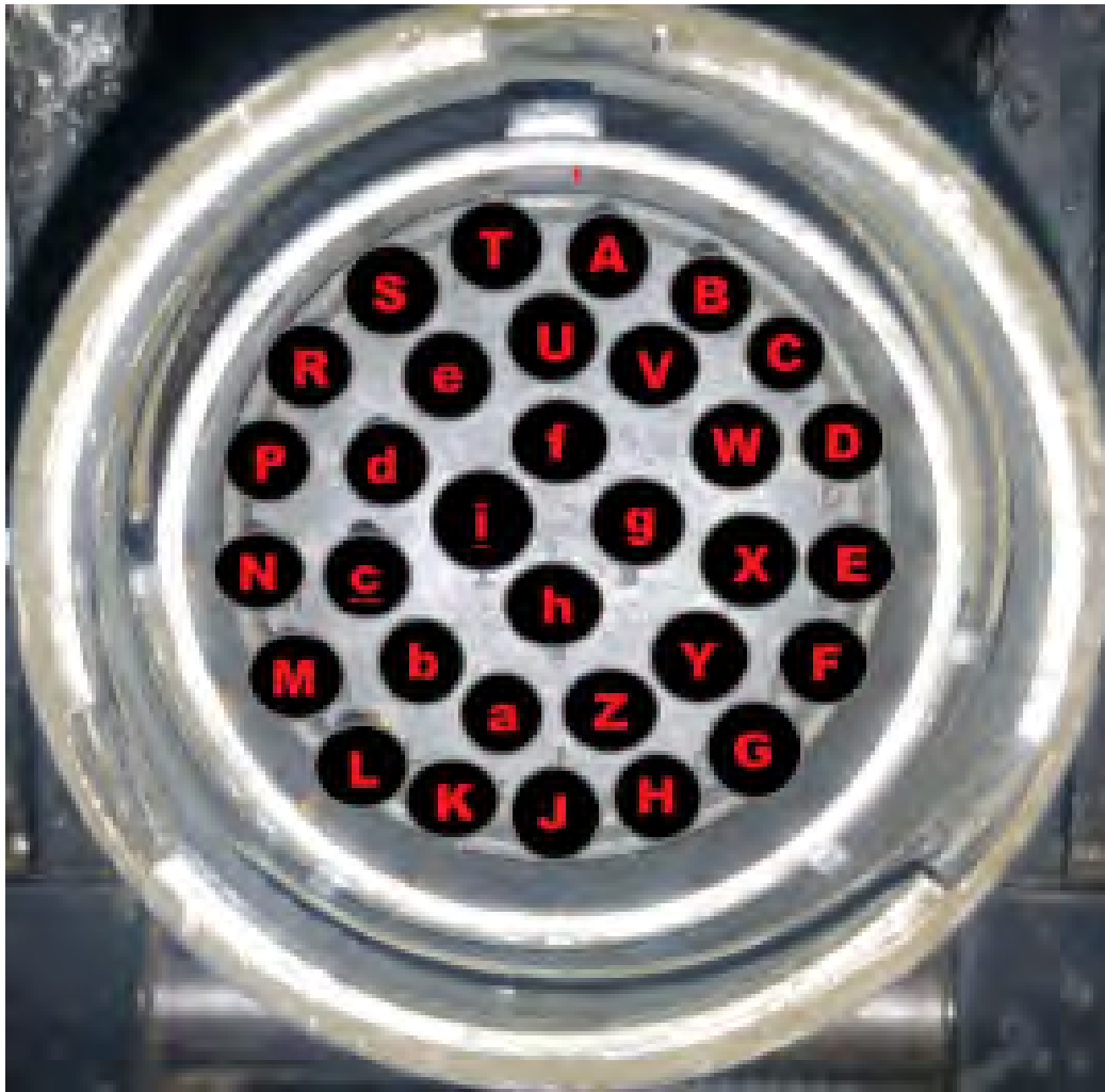
Figure 9.23: Display of the naming convention used to determine the location of pins within each cable.
