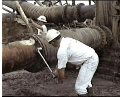
Pushing on a socket wrench may result in forceful exertions near one's maximum capacity.
