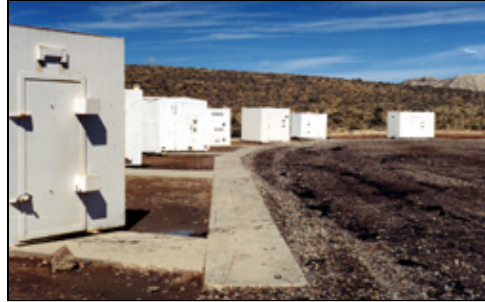
Magazine sidewalks eliminate the uneven walking surfaces while moving blasting supplies.
