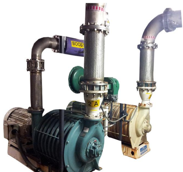
CO2 Booster Compressors at MillerCoors in Golden
