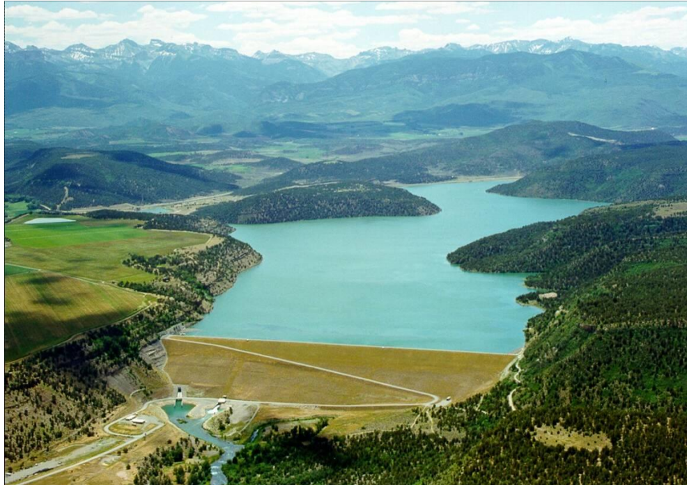
Figure 2: Aerial view of Ridgway Dam.
