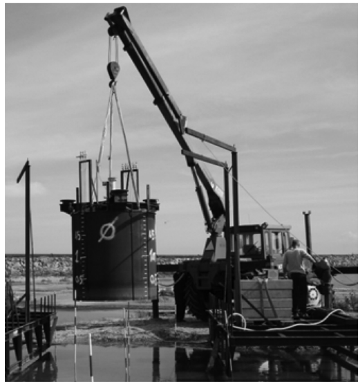
Figure 5. Steel bucket used for the experiments. (The two steel structures at each side of the bucket are used to measure the displacements during loading).
