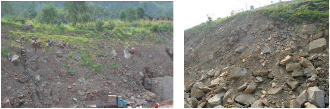
Figure 1. Typical in-situ RSM of Shuima highway project.
